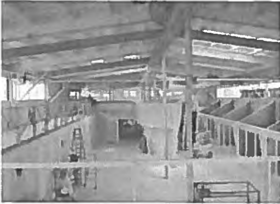
View from mezzanine
