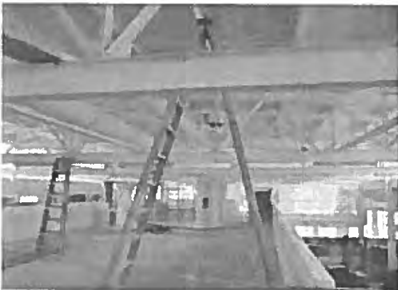
Second floor mezzanine
